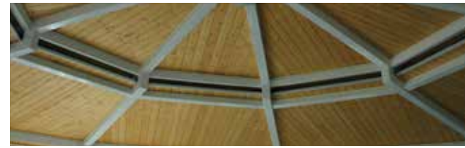
Interior view of Vented Roof Option
